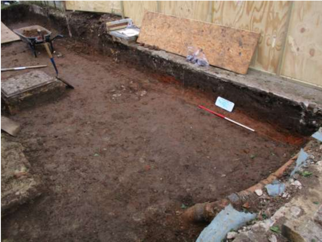
Plate 4. Excavation of the foundation ring beam on the NE area of the site
